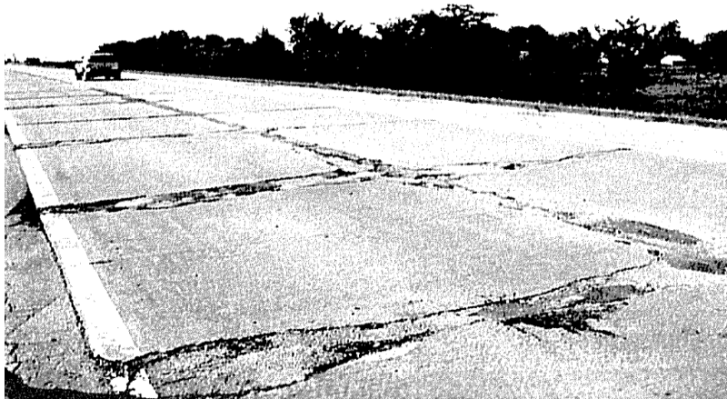
An example of concrete pavement condition in US
